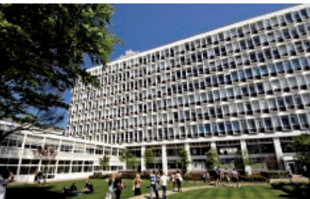
▲ Cockcroft Building, Moulsecomb campus, Brighton.
