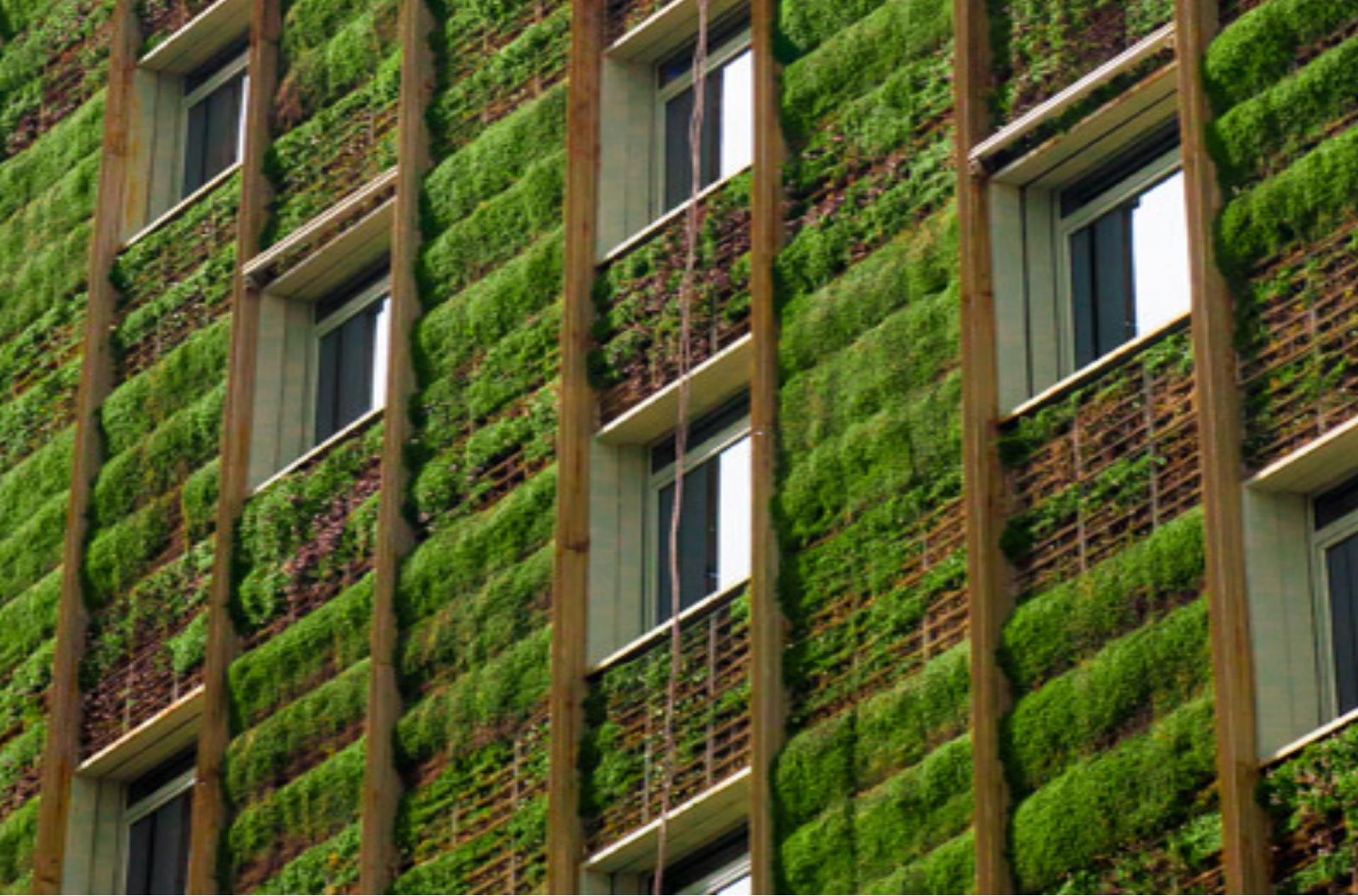
Vegetation growing on a multi-story building
