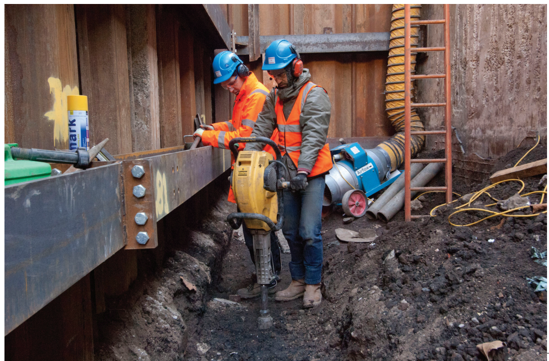
Figure 13.4: Drilling auger holes at the northern perimeter of the site during early phases of excavation 2011–12
