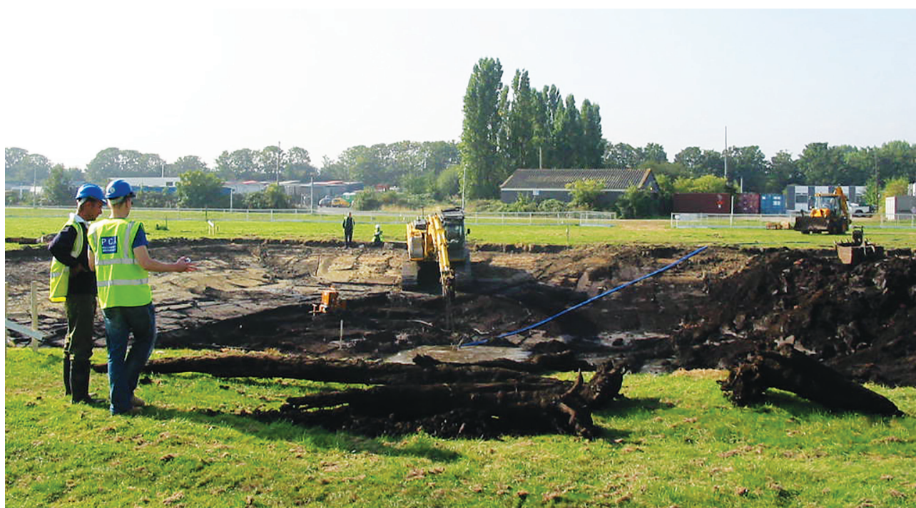
Figure 17.3: Machine 'open-cast' excavation of peat deposits, Crossness Sewage Treatment Works, Bexley (September 2007). Photo courtesy of Historic England
