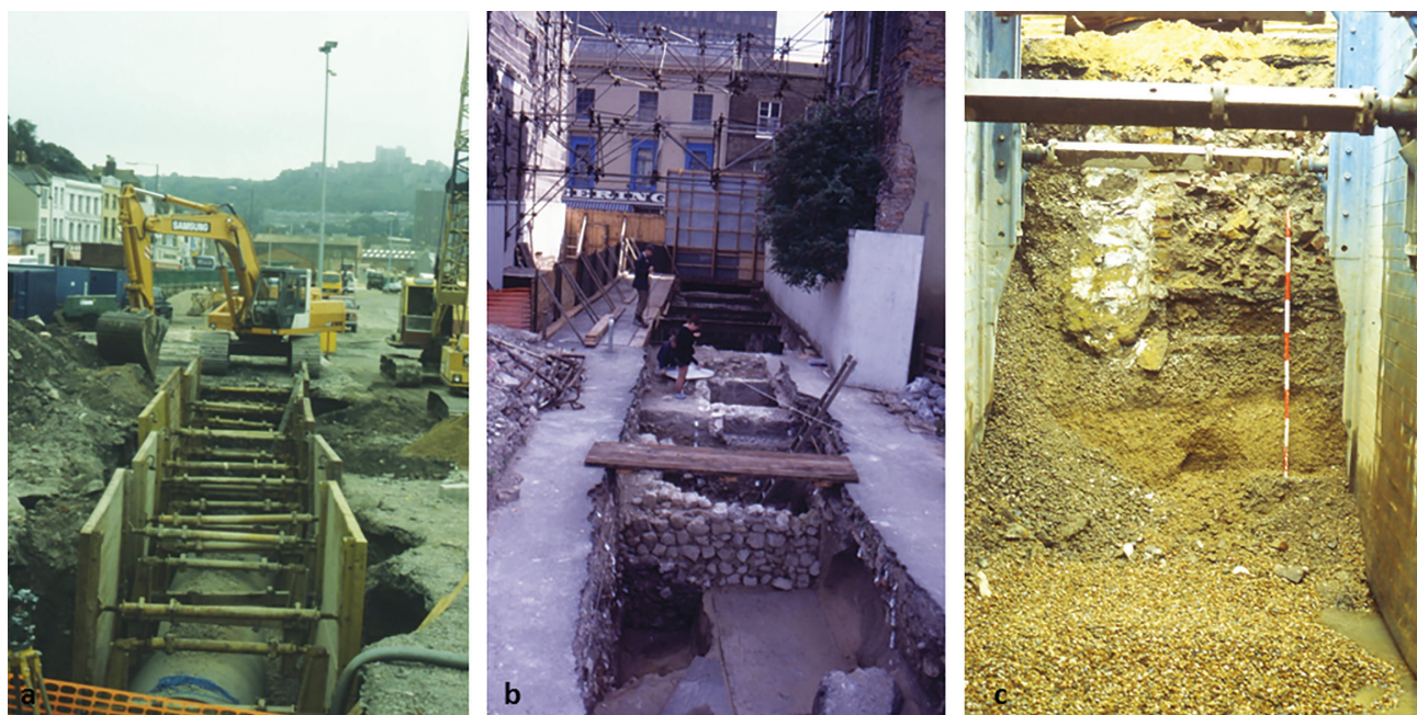
Figure 2.7a: View of sewer trench under excavation. Figure 2.7b: Excavated site. Figure 2.7c: End of trench for recording protected by trench boxes. All photographs by the author
