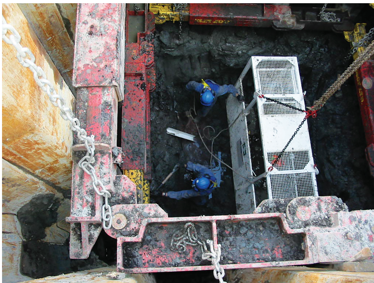
Figure 17.2: A combination of long-reach machine and hand excavation within a shaft to the base of the peat, Belvedere Power Station site, Bexley (October 2007). Photo courtesy of Historic England
