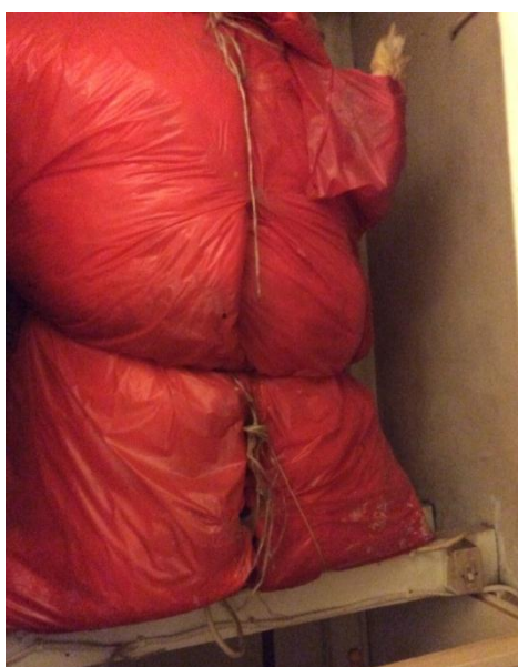
Insulation of water cylinder poor
