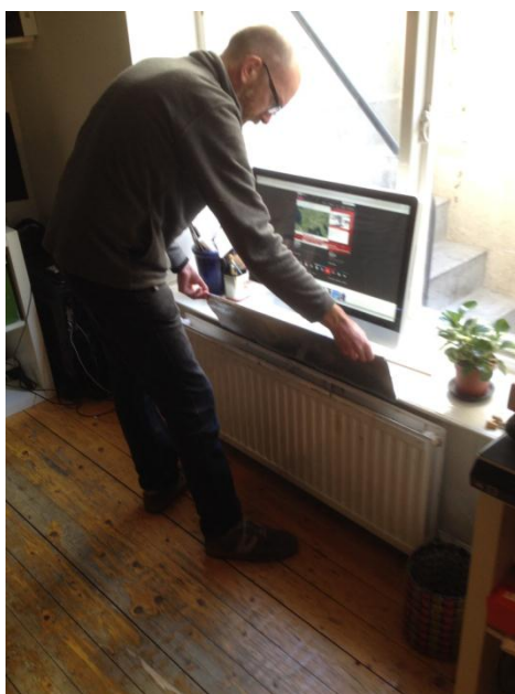
BHESCo installing radiator reflector panel
